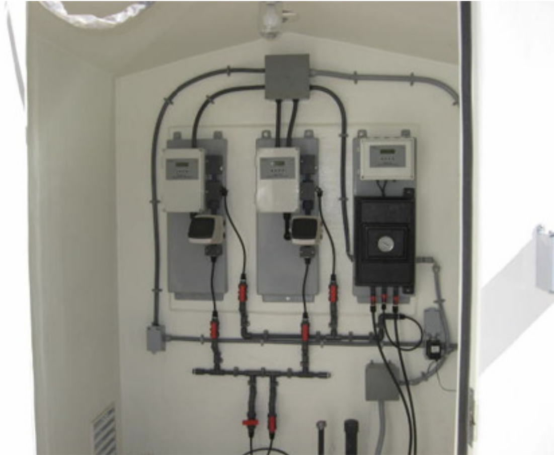
Reliant Water Technologies wastewater chemical disinfection feed system with built-in automatic injector switchover controller and secondary feeder
