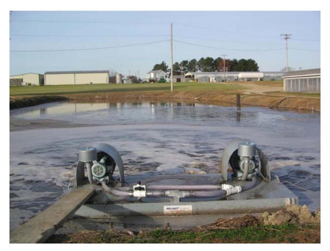
Figure 2: Reliant Model WQA Water Moving Aerator located in one end of the hog lagoon. Photo was taken approximately 15 days after aerator startup.
