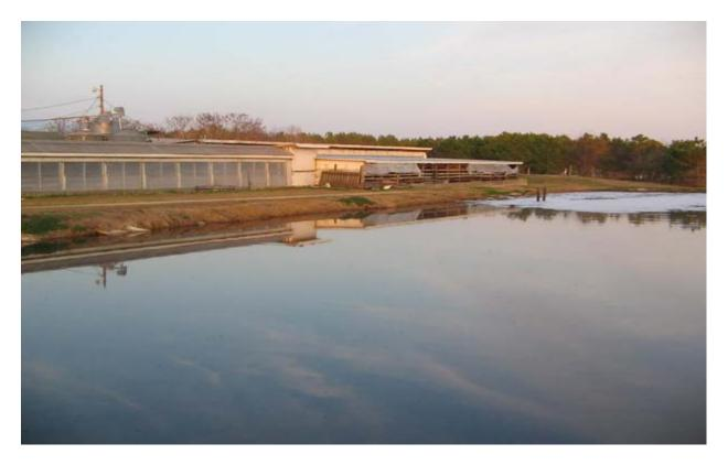
Figure 3: Appearance of the hog lagoon after 60 days of the trial. Note that no sludge is breaking the surface and that all shoreline sludge and foam are no longer present.
